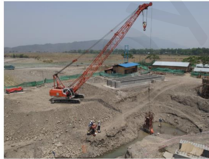
Pile Dynamic Load Test
