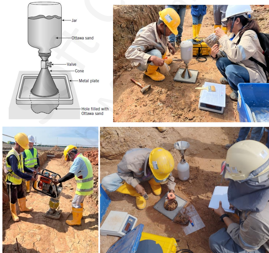
Figure 83: Sand Cone Test Equipment
