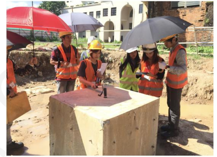
Pile Integrity Test
