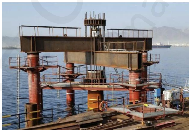
Figure 20: Pile Static Axial Tension Load test
