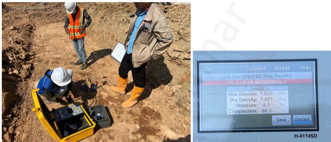
Figure 23: Performing Soil EDG Tests
