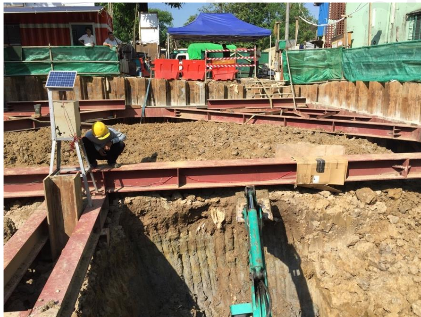
Figure 33: Struct Force Monitoring Station @ Deep Excavation Site
