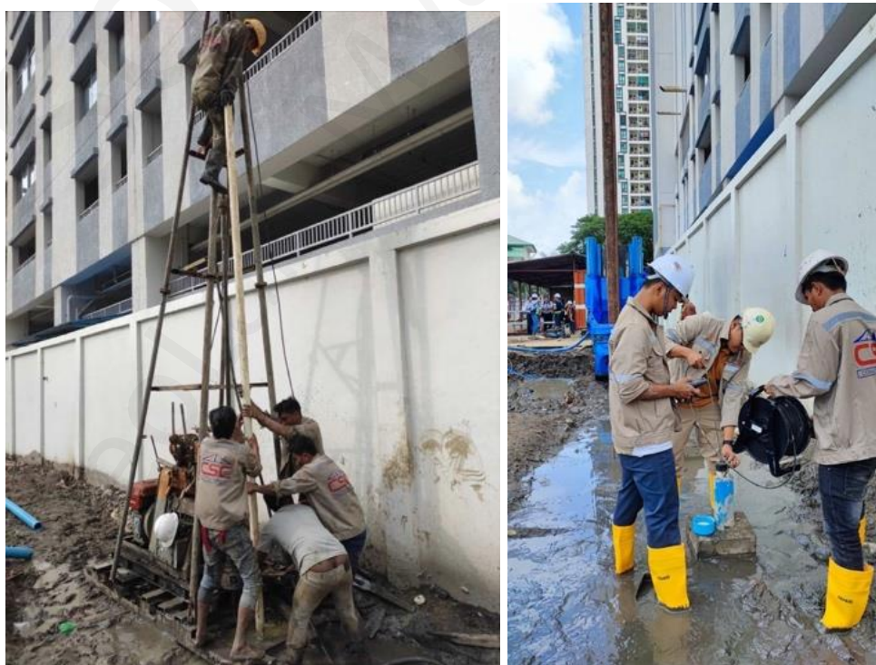
Figure 25: ERSS, TERS, Inclinator Casing, Monitoring
