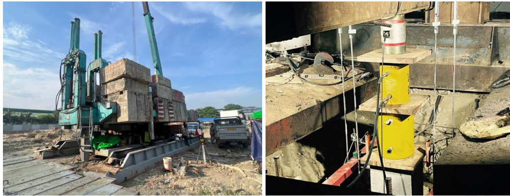
Figure 19: Piling Machine as a Kentledge Counterweight
