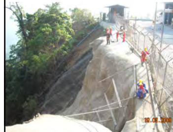
Landslide Repair LSMS1, TEPM, Contractor Teroka-Java Soil Nail + Netting + Guniting (500 sq-m) 20 Dec. 2009 to 20 Mar. 2009 (including pull out test period) 30 Days earlier than schedule
