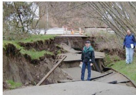
Slope failure by “lateral spreading”
