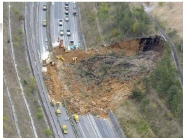
Slope failure by “sliding”
