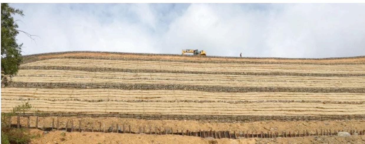
**COMPLETION OF GABION RETAINING WALL (R-1)**
