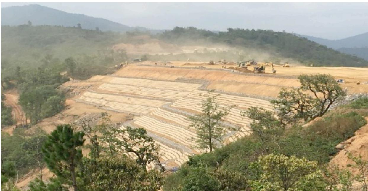
**UNDER CONSTRUCTION STAGE OF GABION RETAINING WALL (R-2)**
