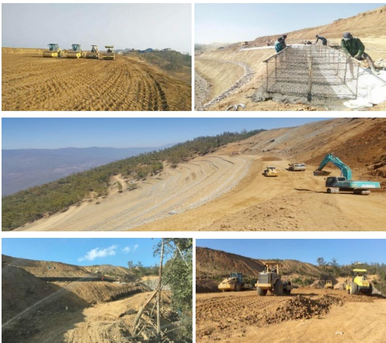
Filling, Spreading, Compacting, Slope and Berm Formation, Gabion Placement & Rock Filling
