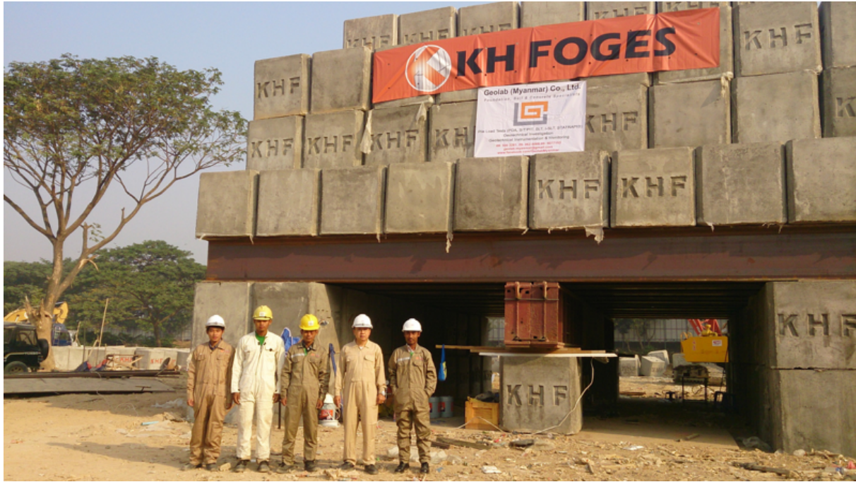
STATIC PILE LOAD TEST WITH KENTLEDGE SYSTEM
