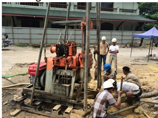
Methods range from non-intrusive geophysics through to fully intrusive borehole installations. The method depends on parameters such as depth, soil type and access to the site. It is common for investigations to be phased - allowing the results of the early phases to guide the next stages.
